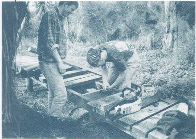
Conservation Corps members rebuild a walkway at Carter's Reserve, Wairarapa.
