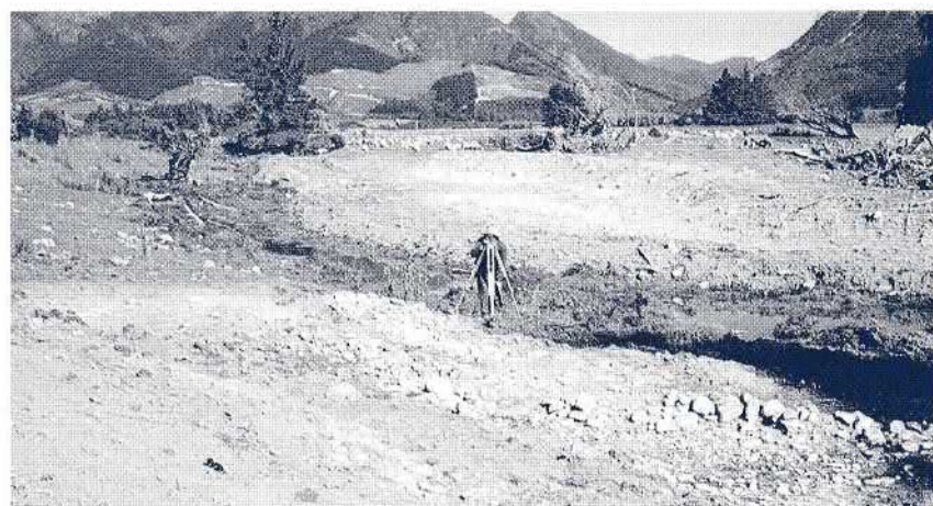
Bill Booth taking levels for the dam wall. Photo Graeme Marshall.
