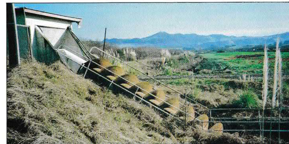
Our Wetlands are being screwed. This archimedes screw pump on the Maramarua sucks 470 million litres a day down the drain. Photo: John Dyer.
