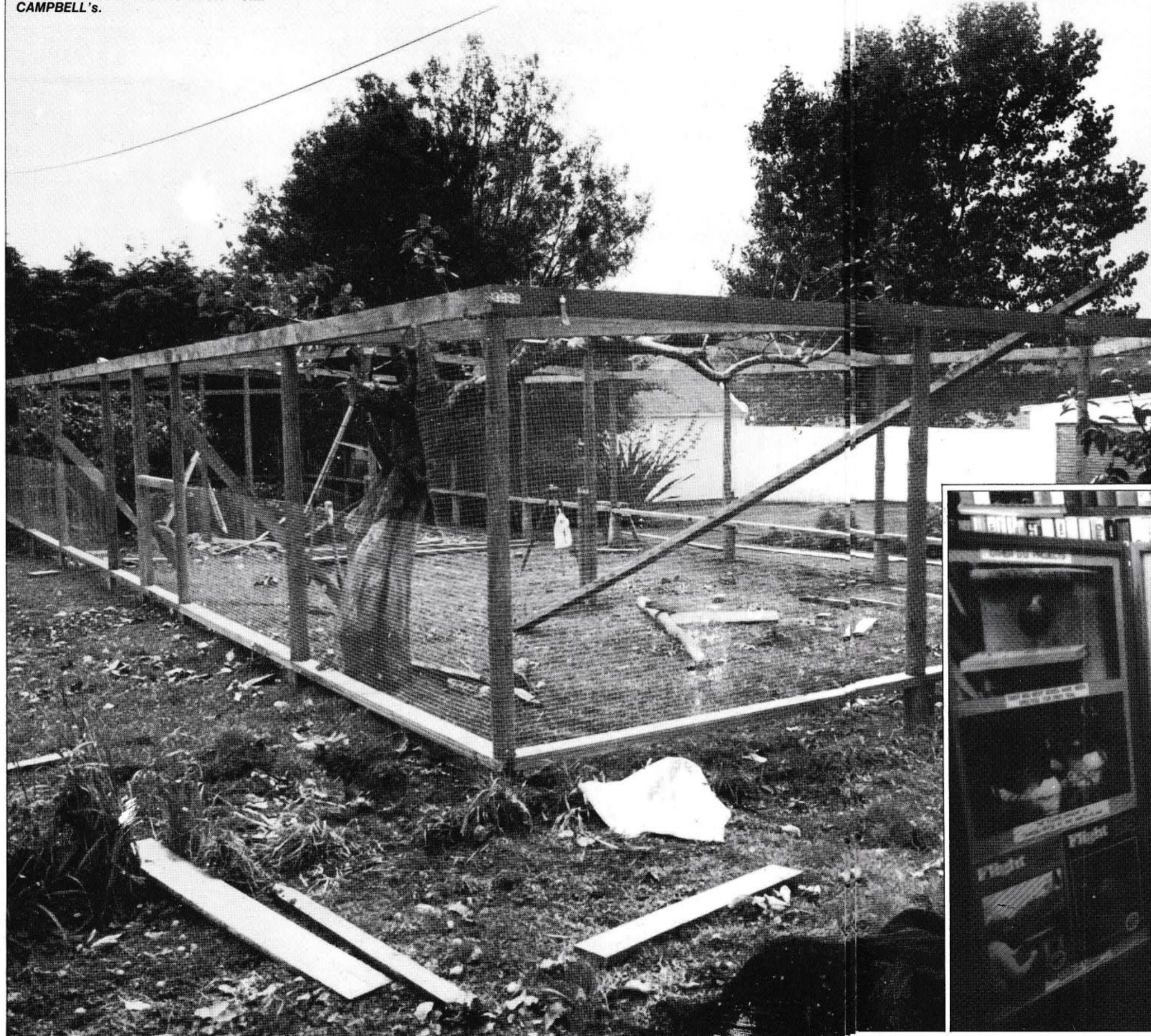
THE BROWN TEAL HOLDING AVIARY UNDER CONSTRUCTION AT JIM CAMPBELL'S.
