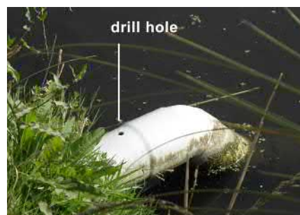
The 45-degree pipe to submerge the inflow – with the later addition of a drill hole and, below, the ‘waterworks’ pipe where a large crack was found, the likely result of the 2014 Eketahuna earthquake.
