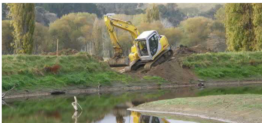
Cutting through the head of the big pond to remove the cluster of rocks.
