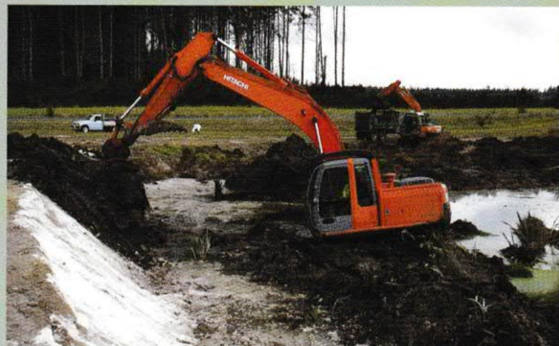
Cover up: Lime covers the pumice and the diggers are putting mud onto the lime. Photos: Jim Campbell.
