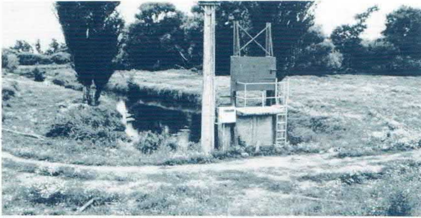
Control gate on a stream flowing into the Waikato River.
